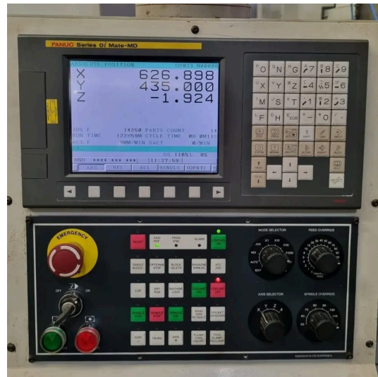
Figure 1. A Fanuc Series oi Mate controller. No user accounts. No password prompt. No access control list.
